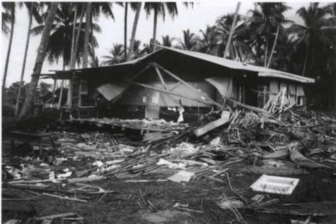
BELOW: The two-storey classroom building was transported 55 m by the wave and came to rest against coconut palms (left). The lower storey of the building collapsed. The view is to the west, October 1998.
